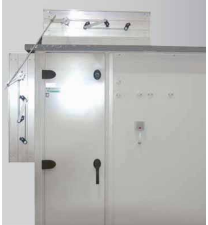
Coupling rod for dampers
