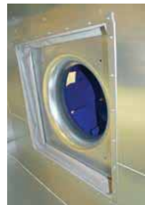
M0 fire class fan flexible connection
