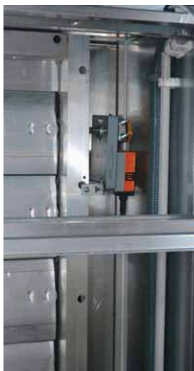
Internal or external damper actuator
