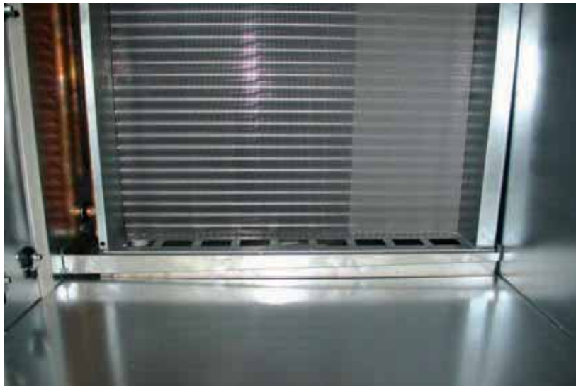
Sloped drain pan
