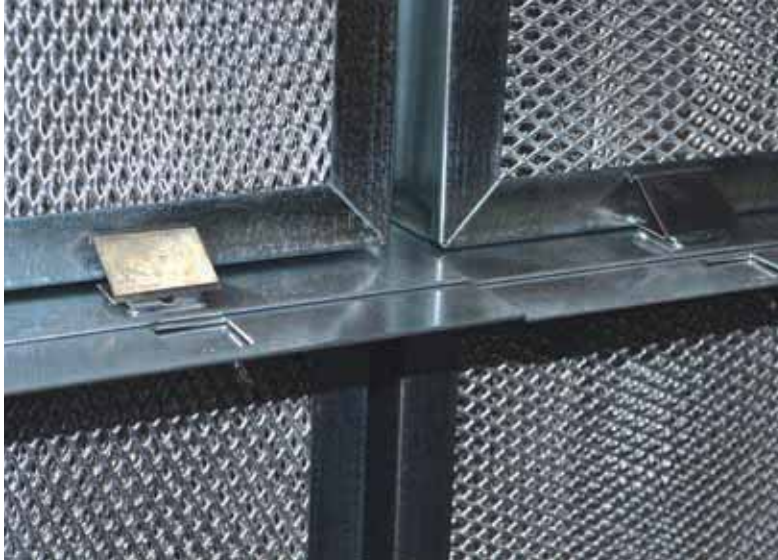
Tightening clip for front withdrawable filter
