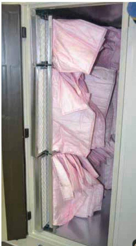
Side withdrawable combined filter (panel + bag)
