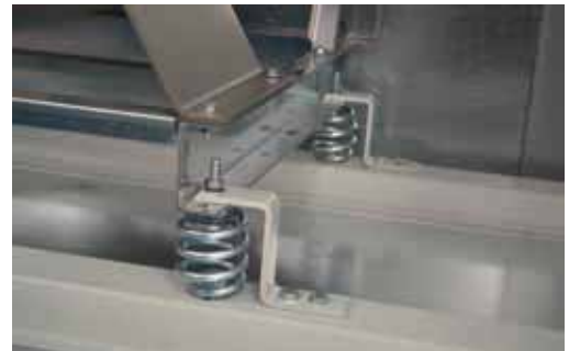
Spring anti vibration mounts
