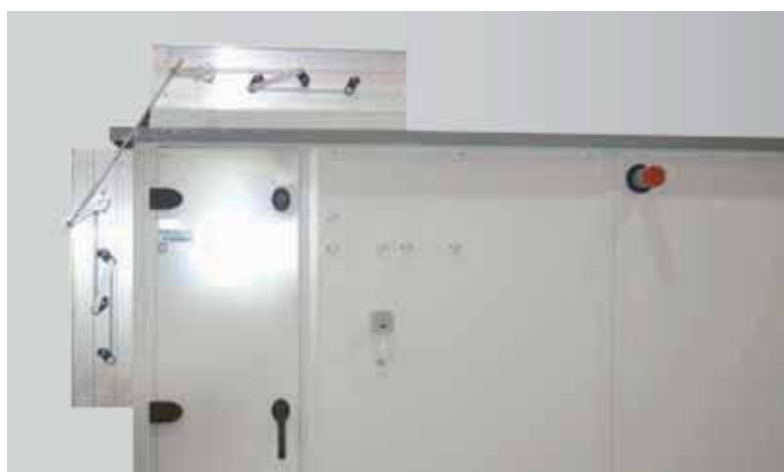
Coupling rod for dampers
